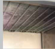
Evaporator freezing shelves provide constant temperature in each compartment.
